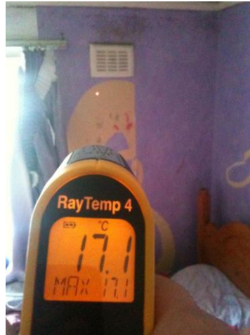
The cavity has been filled
