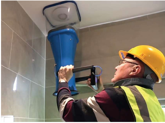
Example of Air flow testing equipment
