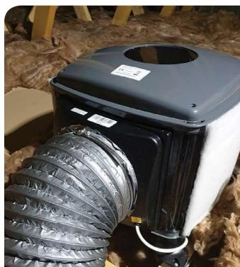
Examples of Positive Input Ventilation
