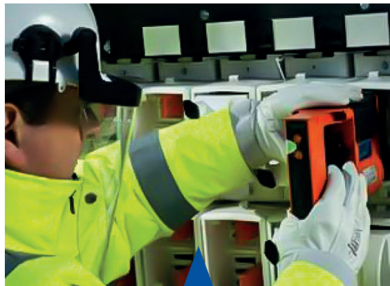
FIGURE 3 – Checking safety before inserting 'J' Type Fuse
