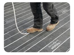
The new low-profile system boasts a lightweight construction, weighing in at a total of 1.2kg per board allowing Craig to effortlessly carry four boards at a time up to the 1st level of the house with ease, compared to the traditional heavier Overlay<sup>™</sup> which weighed 10kg per board.
