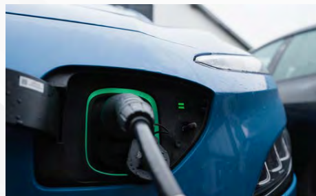
Electric vehicle charging infrastructure
