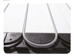
When approaching this renovation, John drew on his wider construction experience and knew exactly what heating system the boat required. John chose Polypipe's Overlay<sup>TM</sup> system, which could be fitted directly on to the boat's floor deck, whilst adding just 18mm in height. John then laid a handmade low profile ply kaboon floor, which is specially made for boats. The two together provided the perfect solution for when ceiling height is at a premium.
