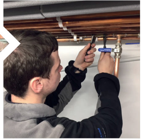
03 Always check and install the bypass and check valves as shown in the manufacturer's installation guide
