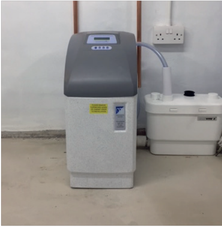
01 Site the softener close to rising main, drain facility and electric supply, allowing access for future servicing and salt replenishment
