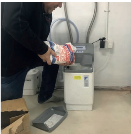
07 Ensure high efficiency of the softener by filling the softener with ultimate tablet salt to within three to four inches of the lid fill point
