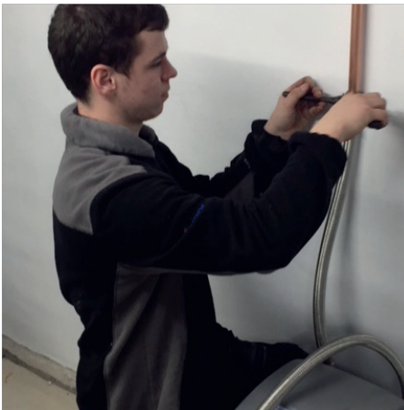
04 Connect the inlet/outlet, overflow and drain hoses to the rear of the softener
