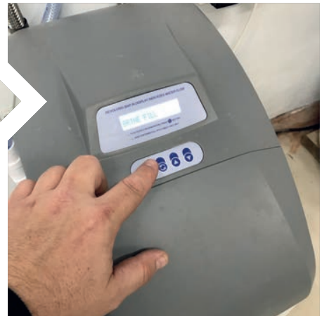
06 Follow the easy to use settings to set the correct water softener hardness level and time using the electronic controller
