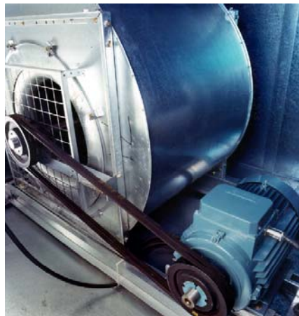
Figure 3 - Belt driven fan assembly
