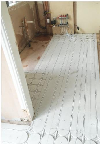
To fit the system, the underfloor heating pipes (12mm Multi-Layer Composite Pipe) are laid within the 18mm thick pre-routed Overboard panels, offering a low profile solution which lends itself to situations where minimal floor height adjustments are desired. This makes the Overboard system suitable for virtually any property desiring underfloor heating with its indoor comfort benefits, lower heating bills and reduced CO<sub>2</sub> emissions.
